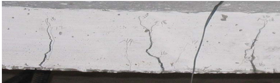
Figure 5: Photograph of cracks propagation
