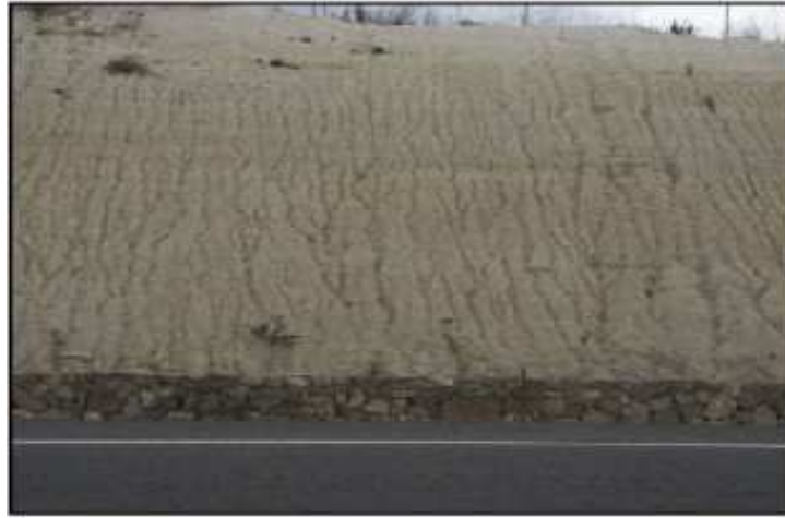
Figure 1. Newly constructed embankment [2].
